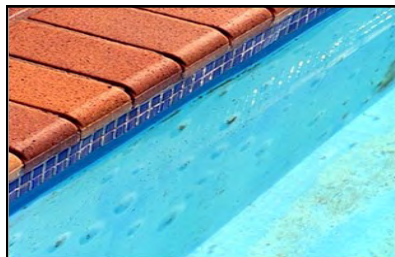
Osmosis in a fibreglass pool
